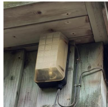
E209: External lighting diffuser degraded.
