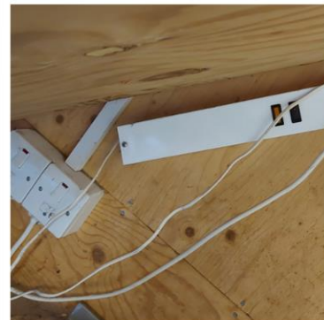
E206: Final circuit cables not supported.
