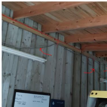
E205: Final circuit cables not supported.
