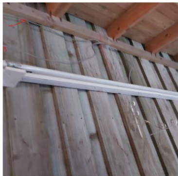
E204: Final circuit cables not supported.
