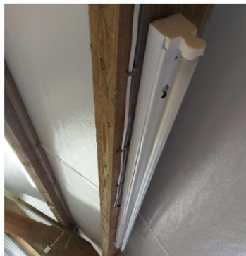
E207: Internal lighting missing diffuser and not working.
