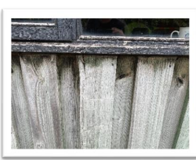
B105: Externally the timber sills and timber cladding below the sills are showing signs of damp and rot
