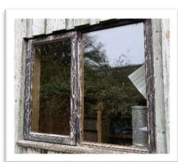
B104: External windows are showing signs of minor rot, water ingress and heavily weather externally
